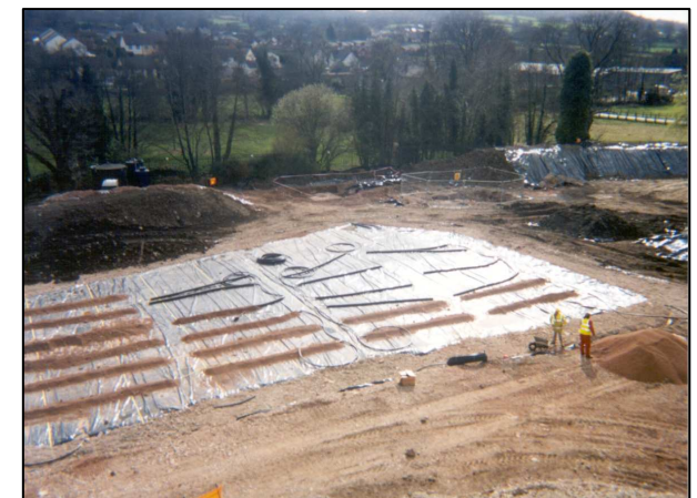
Photograph 2: Preparation of biopile treatment area
