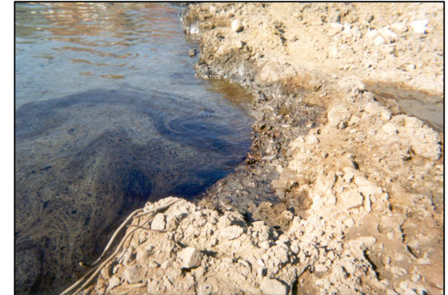
Photograph 1: Floating free product in open excavation
